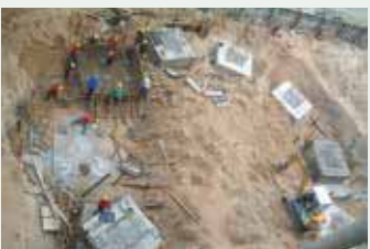
Construction of Spherical Tank Foundation
