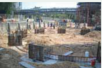
Foundation of Spherical Tank
