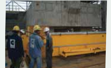
Over Head Crane Installation
