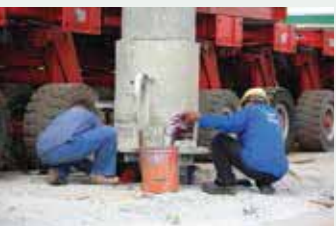
Foundation of Spherical Tank
