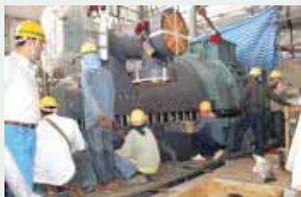
Installation of Steam Turbine Generator
