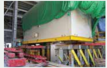
Skidding & Jacking of Steam Condensor
