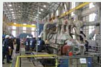
Installation of Steam Turbine Generator
