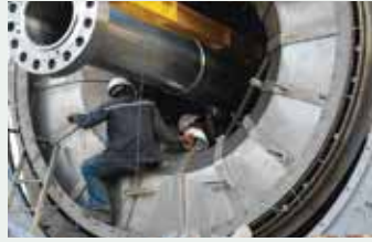
Installation of Gas Turbine
