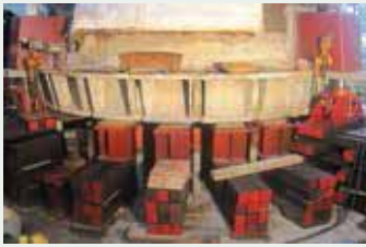
Special Work - Rotate EB/SM Reactor (200 tons)
