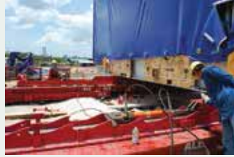
Skidding & Jacking of Gas Turbine
