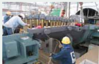
Installation of Steam Turbine Generator
