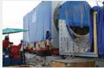
Installation of Gas Turbine
