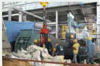
Installation of Steam Turbine Generator
