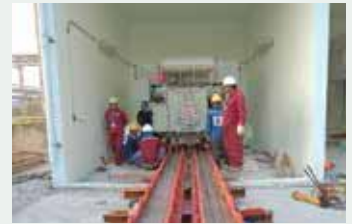
Skidding & Jacking of Steam Condensor
