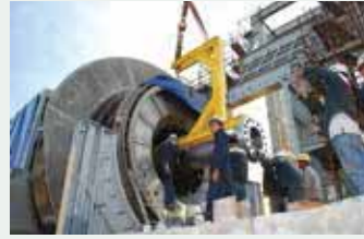
Installation of Gas Turbine
