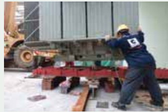
Skidding & Jacking of Transformer
