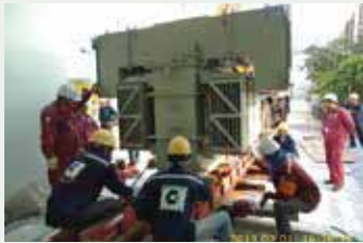
Special Work - Rotate EB/SM Reactor (200 tons)
