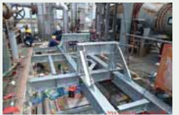
Installation of Structure for Equipment Installation
