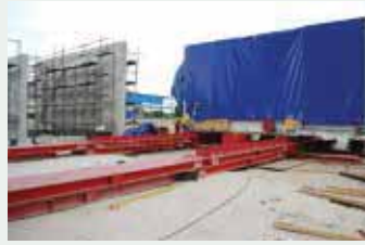
Skidding & Jacking of Gas Turbine
