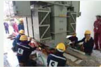
Skidding & Jacking of Transformer
