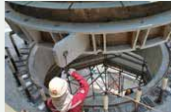
Installation of EB/SM Reactor
